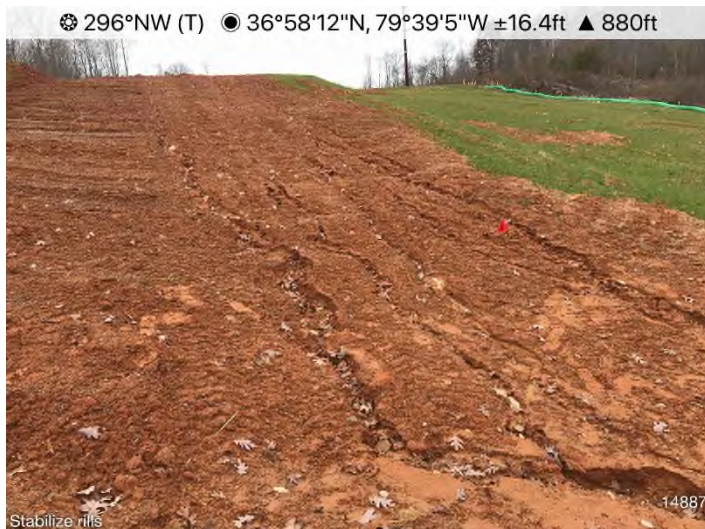
Fig. 3: STA 14861+50 to 14907+50 – Stabilization of travel lane needed.
