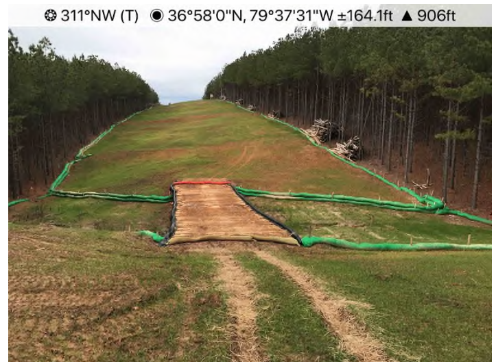
Fig. 4: STA 14960+00 – Controls in place and functioning. Area stabilized with vegetative cover.
