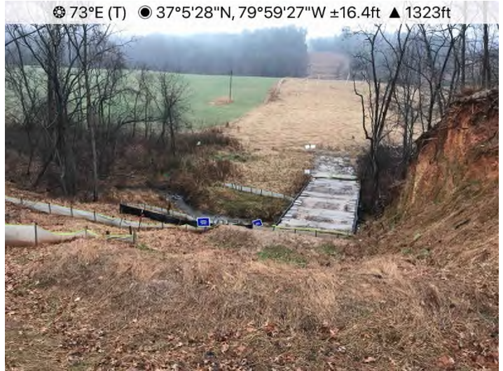
Fig. 4: Stream S-KL36 – Controls in place and properly functioning along Stream S-KL36 crossing.
