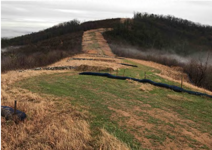
Fig. 3: Stream S-II7 – Controls in place and functioning above Stream S-II7. Area stabilized with vegetation.
