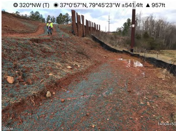
Fig. 3: STA 14504+50 – Erosion control matting needed on steep slope.
