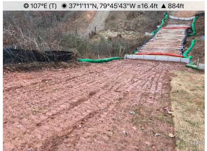
Fig. 4: STA 14486+00 – Stabilization needed on CIS slope of Stream S-G22.
