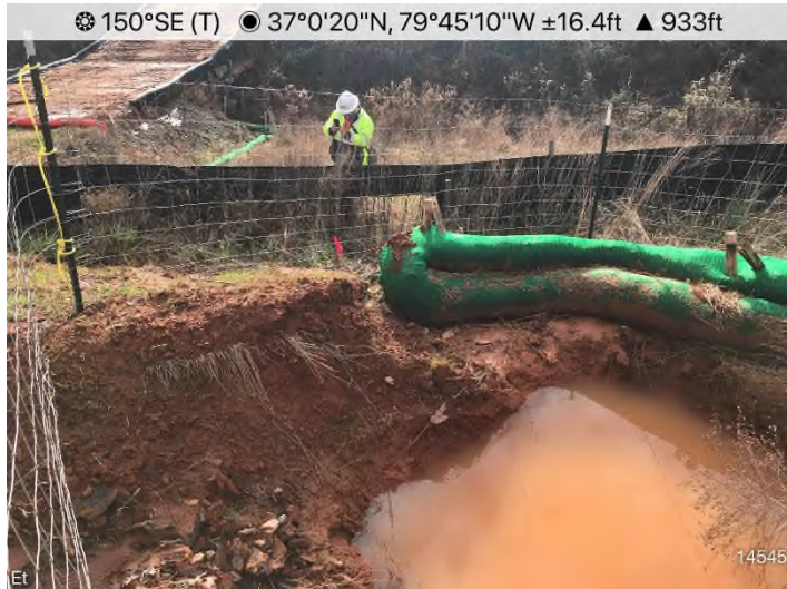
Fig. 3: STA 14504+50 – Erosion control matting needed on steep slope.
