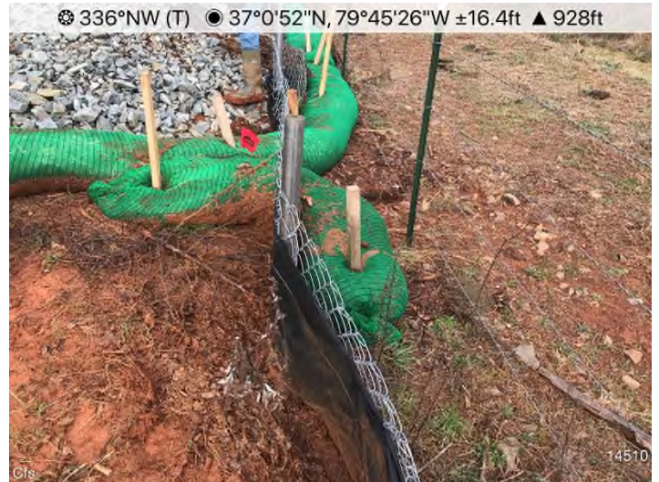
Fig. 4: STA 14486+00 – Stabilization needed on CIS slope of Stream S-G22.
