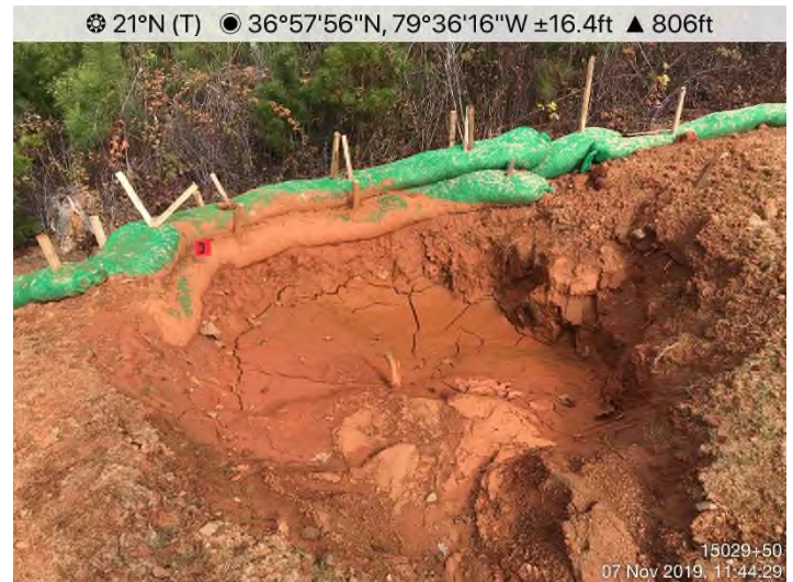
Fig. 4: STA 15049+00 – Waterbar filled with sediment. Maintenance needed.
