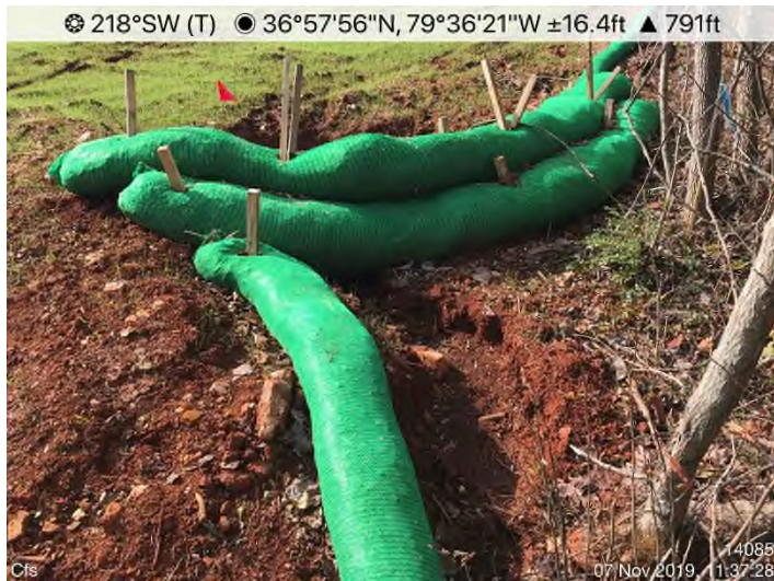
Fig. 3: STA 15047+00 to 15048+00 – P1 undermined in several locations. Maintenance needed.
