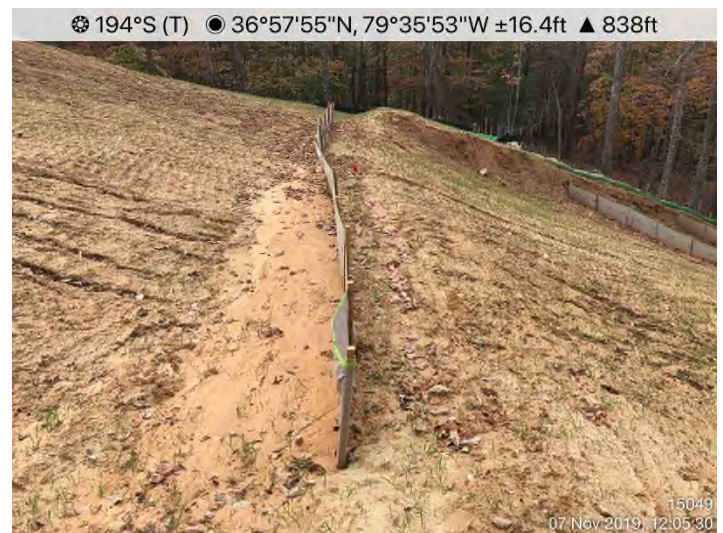
Fig. 4: STA 15049+00 – Waterbar filled with sediment. Maintenance needed.
