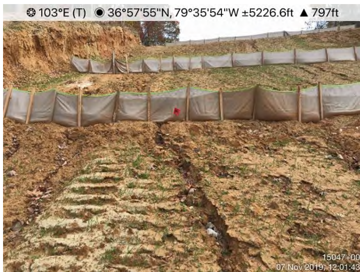
Fig. 3: STA 15047+00 to 15048+00 – P1 undermined in several locations. Maintenance needed.
