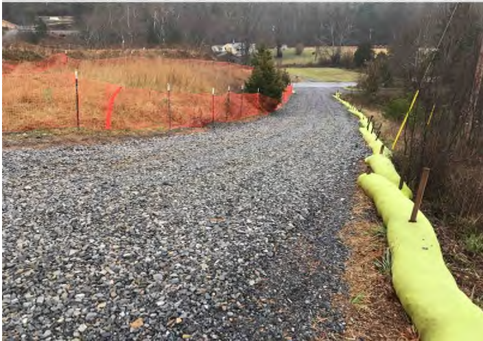
Fig. 3: STA 12183+33 – Controls in place and functioning. Area stabilized with seed, straw and hydro-mulch.
