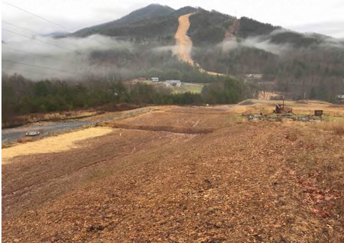
Fig. 3: STA 12183+33 – Controls in place and functioning. Area stabilized with seed, straw and hydro-mulch.
