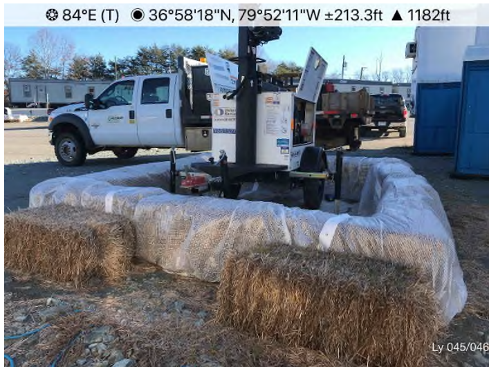
Fig. 3: Laydown Yard 032 – Controls in place. Secondary containment structure functioning properly.
