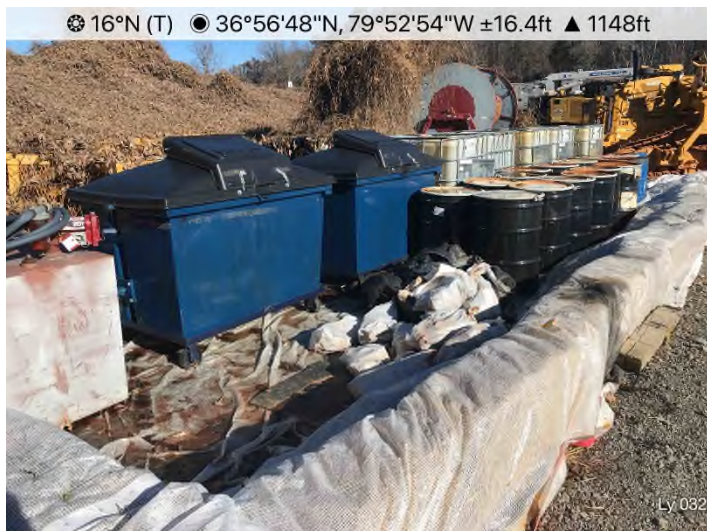
Fig. 3: Laydown Yard 032 – Controls in place. Secondary containment structure functioning properly.
