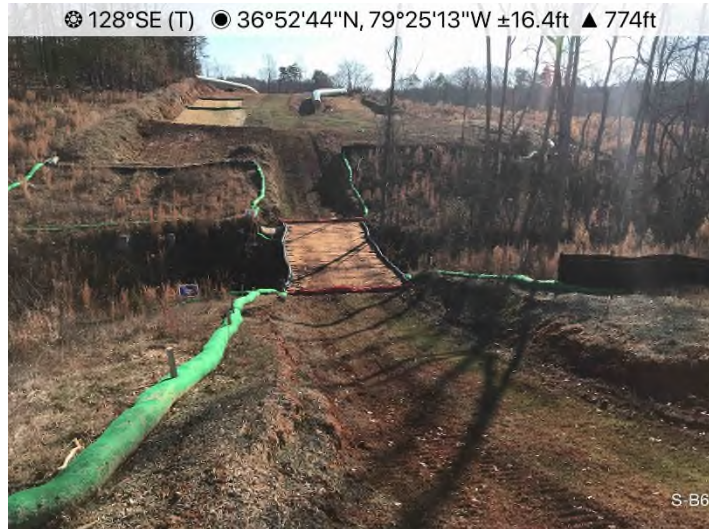
Fig. 3: STA 15795+00 – Controls in place and properly functioning at Stream S-C1. Area stabilized.
