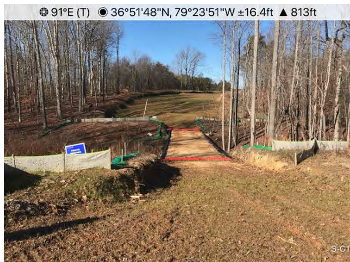
Fig. 3: STA 15795+00 – Controls in place and properly functioning at Stream S-C1. Area stabilized.
