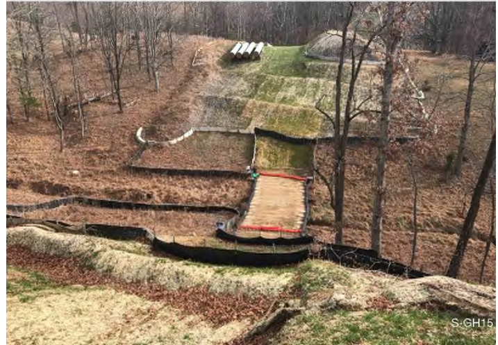
Fig. 4: Stream S-GH15 – Controls in place and properly functioning along stream S-GH15. Area stabilized with erosion matting.
