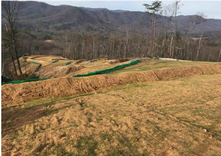
Fig. 3: STA 13371+00 – Controls in place and functioning. Area stabilized with erosion matting.
