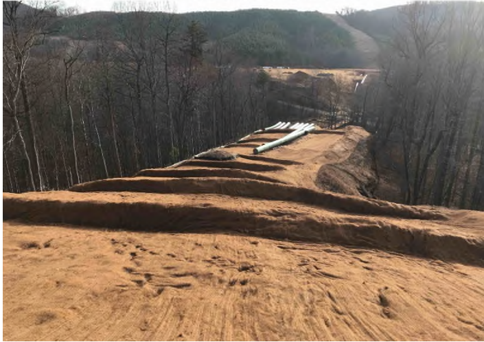
Fig. 3: STA 13371+00 – Controls in place and functioning. Area stabilized with erosion matting.
