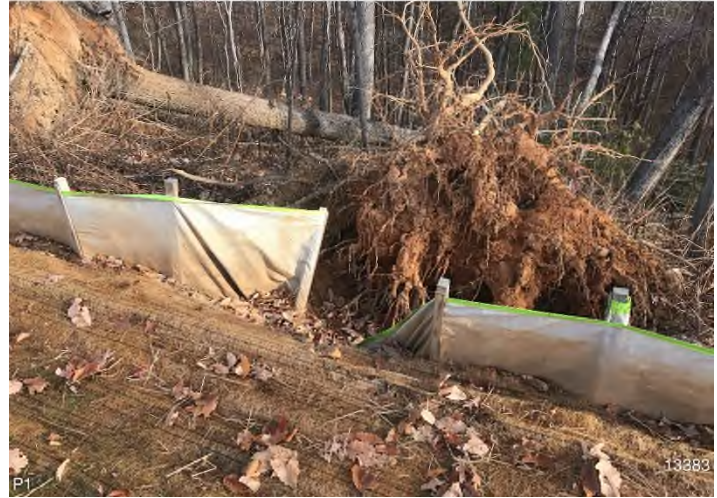
Fig. 4: Stream S-GH15 – Controls in place and properly functioning along stream S-GH15. Area stabilized with erosion matting.
