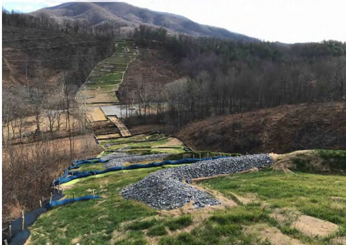
Fig. 3: STA 13254+00 – Controls in place and properly functioning. Area stabilized.
