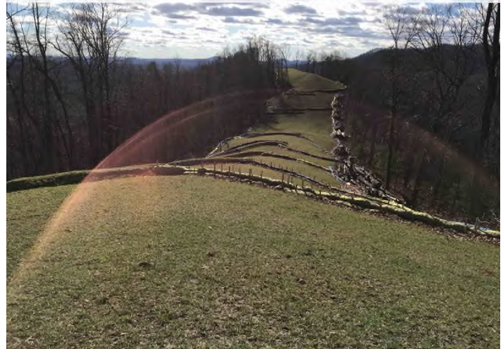
Fig. 4: STA 13230+00 – Controls in place and properly functioning. Area stabilized.
