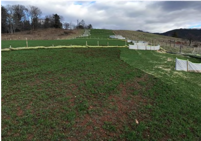
Fig. 3: STA 13254+00 – Controls in place and properly functioning. Area stabilized.
