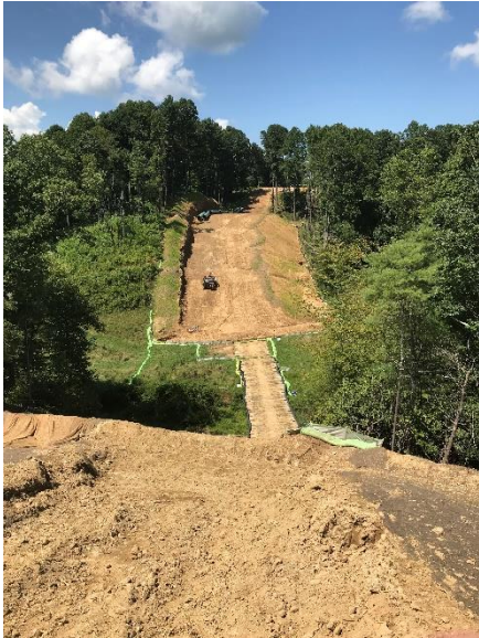
Fig. 1 Near station 13026+00, water bar and stabilization matting installed
