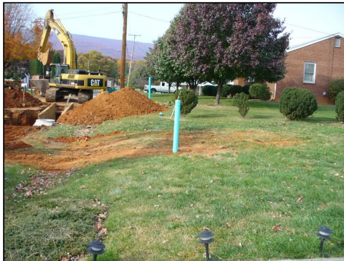
Figure 7.3. Photo showing home with failing septic system being connected to Western VA Water Authority sewer line (Photo: DEQ)
