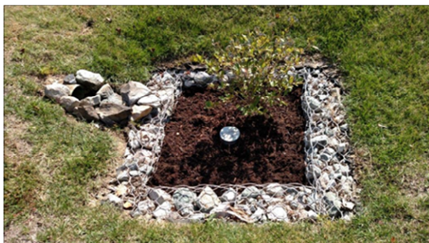
Figure 7.10. Manufactured urban stormwater BMP (Photo: Timmons Group)
