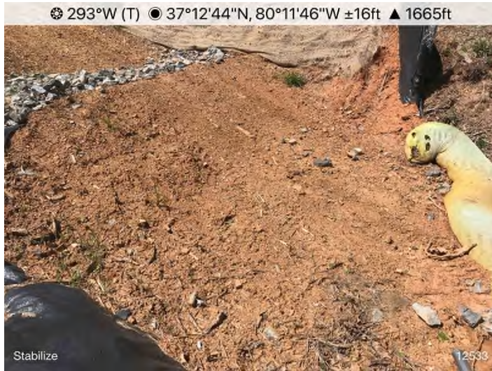
Figure 5: STA 12533+00 – Re-stabilize denuded area for landowner access below checkdam.
