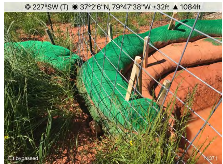
Figure 4: STA 14371+00 – End treatment bypassed.
