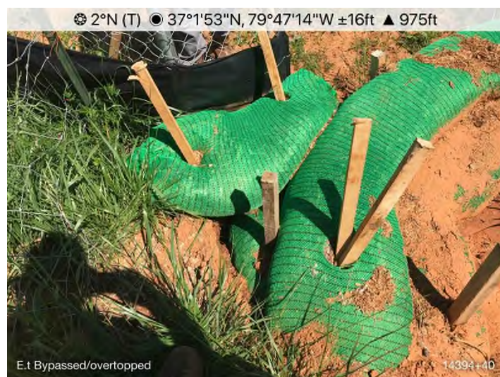
Figure 7: STA 14394+40 – End treatment bypassed.
