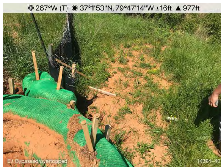
Figure 8: STA 14394+50 – Re-stabilize stockpile in ATWS 623.
