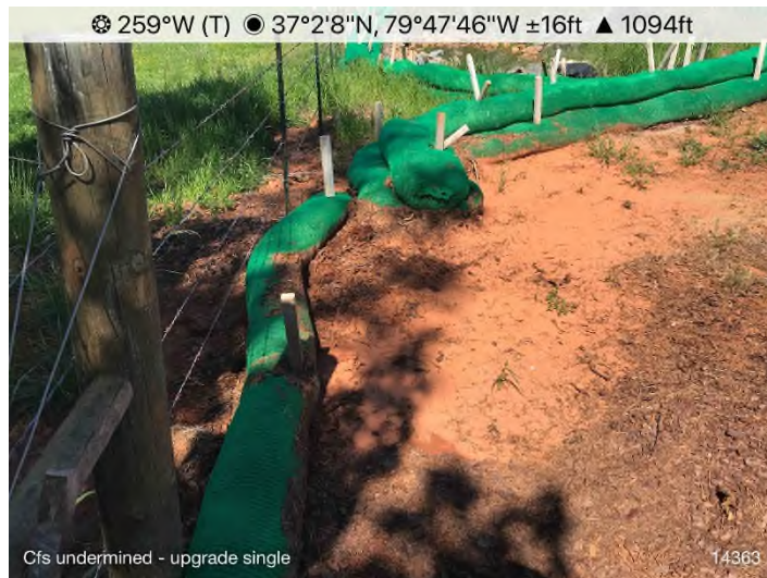
Figure 3: STA 14363+00 – CFS undermined.
