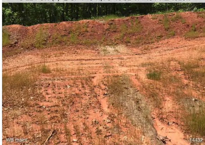
Figure 11: STA 14432+00 – Waterbar maintenance needed.
