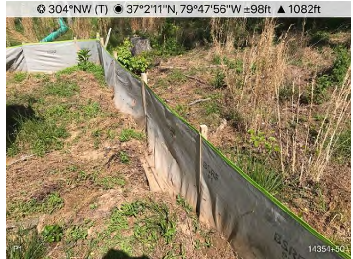
Figure 4: STA 14371+00 – End treatment bypassed.
