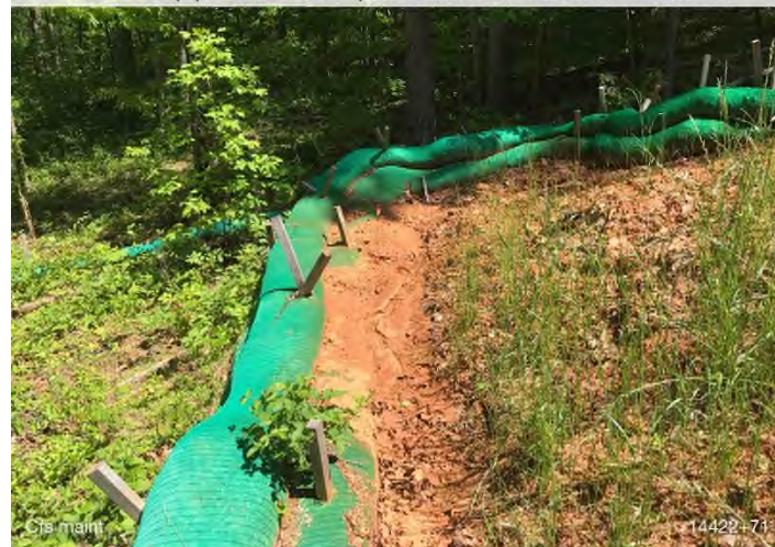
Figure 10: STA 14422+71 – CFS maintenance needed.
