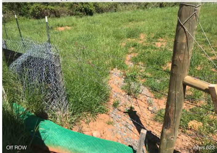
Figure 11: STA 14432+00 – Waterbar maintenance needed.
