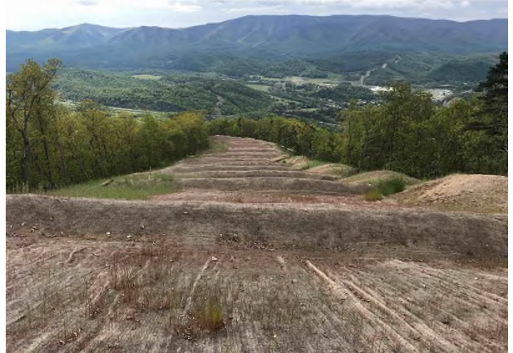
Figure 4: STA 12363+00 – Controls in place and functioning properly. Area stabilized with erosion control matting.
