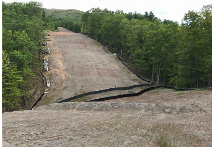
Figure 4: STA 12363+00 – Controls in place and functioning properly. Area stabilized with erosion control matting.
