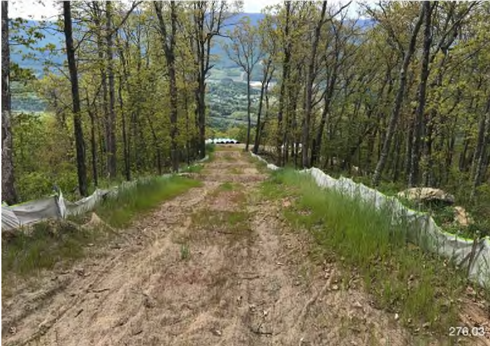
Figure 3: STA 12334+00 – Controls in place and functioning properly. Area stabilized with erosion control matting.
