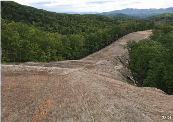
Figure 3: STA 12334+00 – Controls in place and functioning properly. Area stabilized with erosion control matting.
