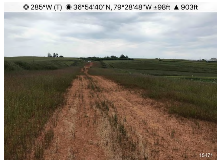
Figure 4: STA 15471+00 – Controls in place and functioning properly. ROW stabilized, no erosion present within travel lane.
