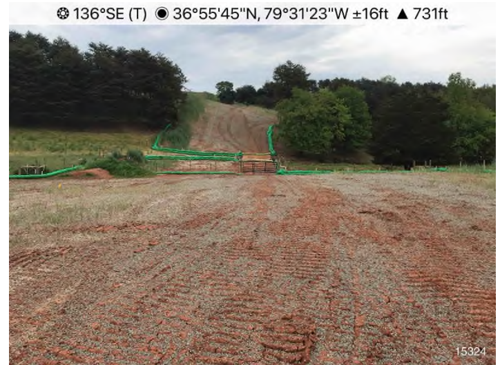
Figure 4: STA 15471+00 – Controls in place and functioning properly. ROW stabilized, no erosion present within travel lane.
