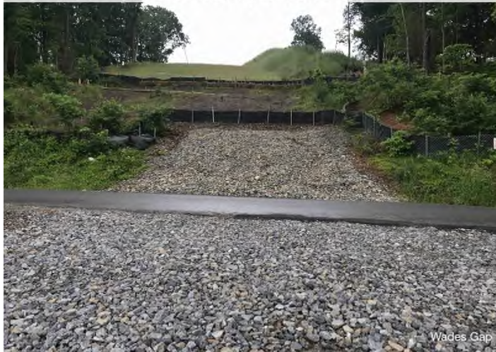
Figure 3: STA 11306+50 – Controls in place and functioning properly at the Cahas Road crossing.
