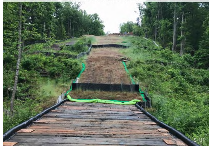
Figure 4: Stream S-IJ1 – Controls in place and functioning properly at stream S-IJ1 crossing. Area stabilized.
