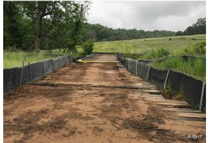
Figure 4: Stream S-IJ1 – Controls in place and functioning properly at stream S-IJ1 crossing. Area stabilized.
