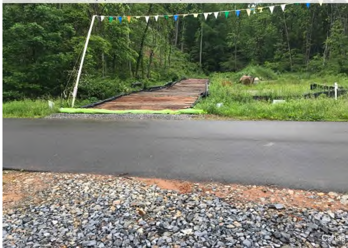
Figure 3: STA 11306+50 – Controls in place and functioning properly at the Cahas Road crossing.
