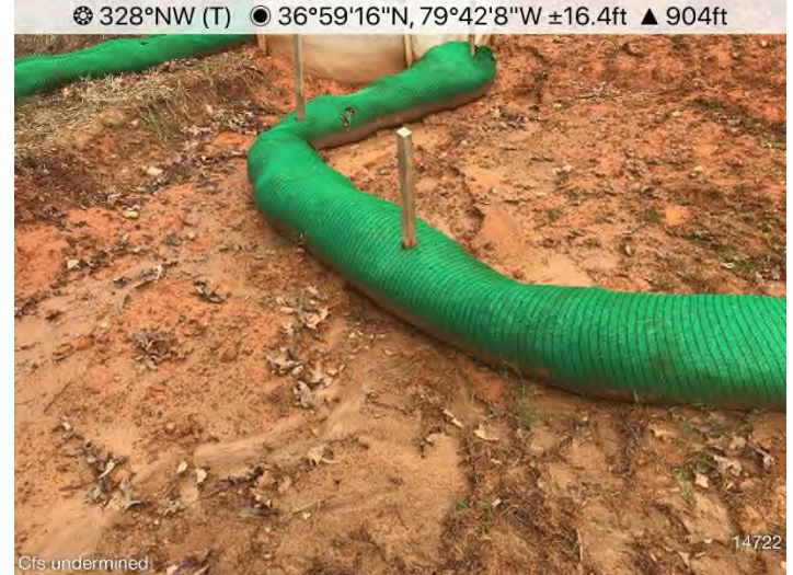
Figure 4: STA 14713+00 – P1 undermined. Repair needed.
