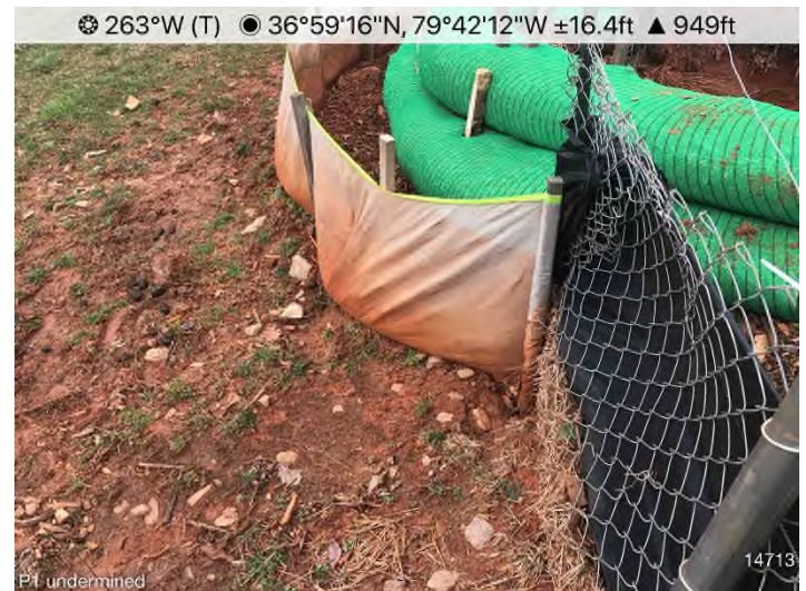
Figure 4: STA 14713+00 – P1 undermined. Repair needed.
