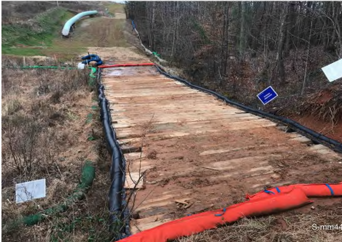
Figure 3: STA 14833+00 – SSF maintenance needed.
