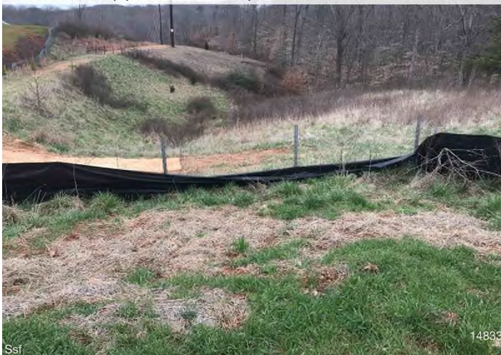
Figure 3: STA 14833+00 – SSF maintenance needed.
