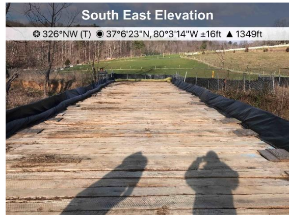
Figure 2: Designated crossing S-GH7, ECD's are in place.
