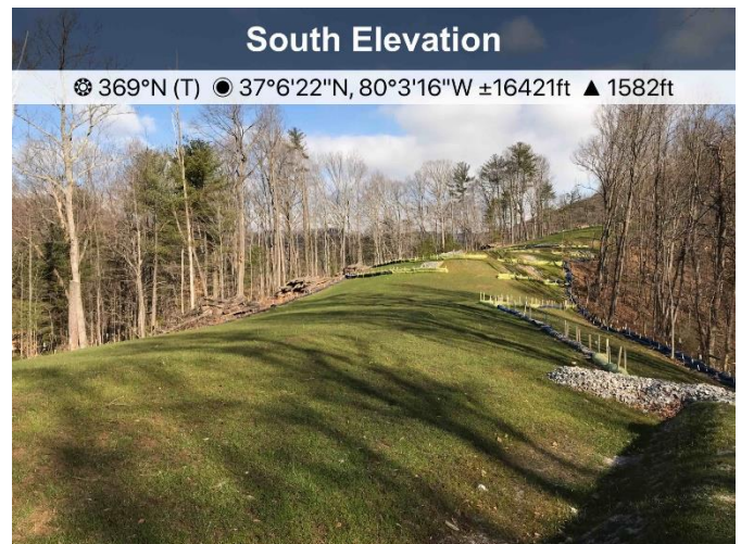
Figure 4: Near MP25.3 ECD's are in place and the area is well stabilized.
