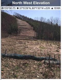
Figure 3: Designated crossing S-IJ4, ECD's are in place.
