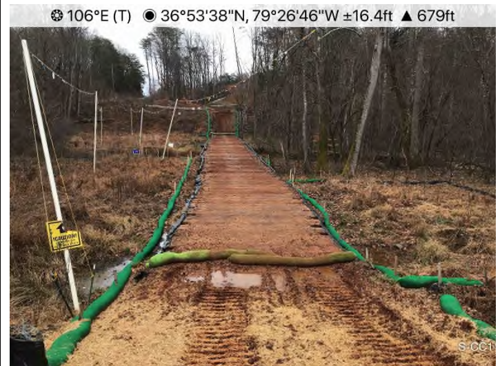
Figure 4: STA 15641+00 – Controls in place and functioning properly. Area stabilized with Earth-Guard.
