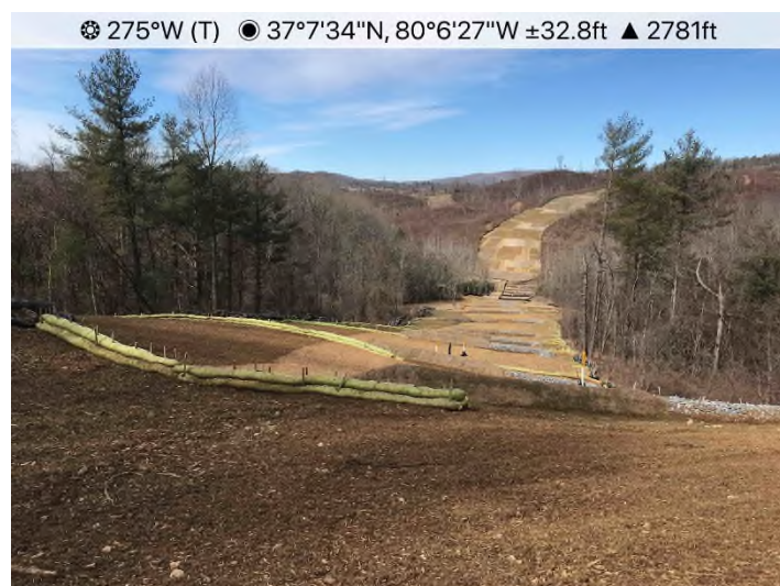
Figure 3: STA 13072+00 – Controls in place and functioning properly.
