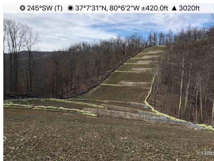
Figure 4: Stream S-G26/27 – Controls in place and functioning properly.
