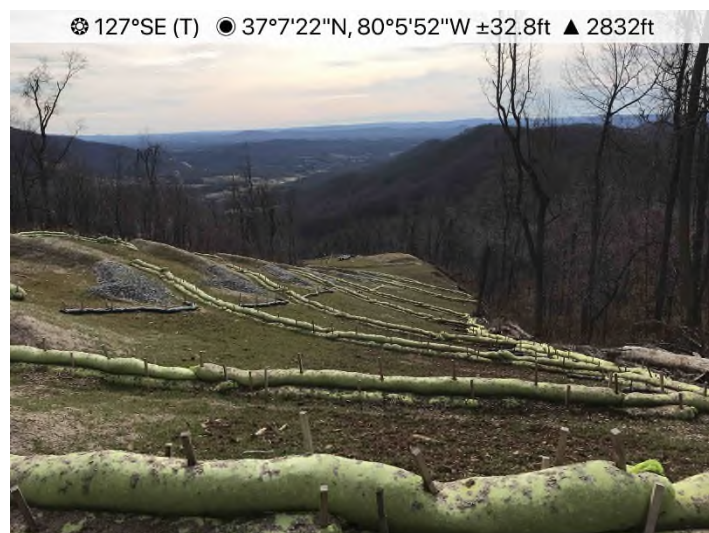
Figure 3: STA 13072+00 – Controls in place and functioning properly.
