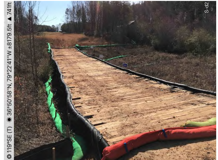
Figure 4: STA 15937+00 to 15939+00 – Re-stabilization needed.
