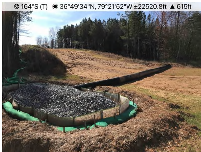
Figure 3: STA 15933+00 – Controls in place and functioning properly.
