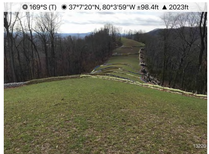
Figure 4: STA 13220+00 – Controls in place and functioning properly.
