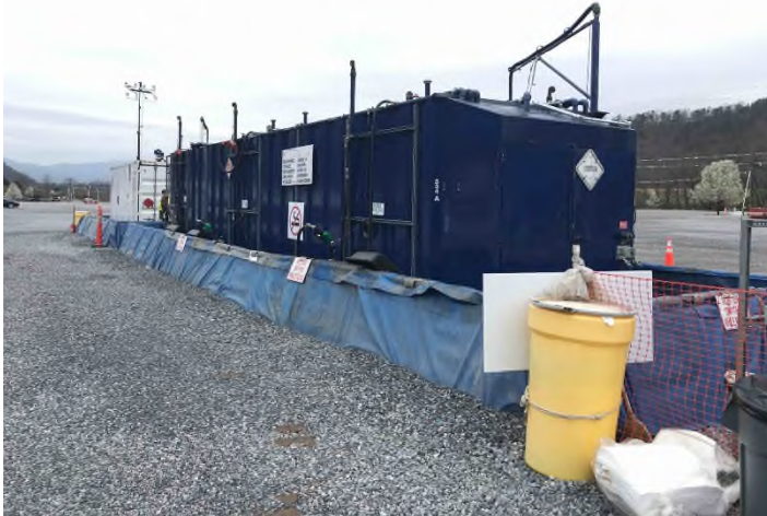
Figure 3: Laydown Yard 049 – Drip pans in place and functioning properly.
