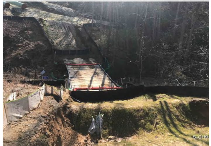
Figure 4: Stream S-GH9 – Controls in place and functioning properly. Area stabilized with erosion matting. No evidence of sediment discharge off ROW.
