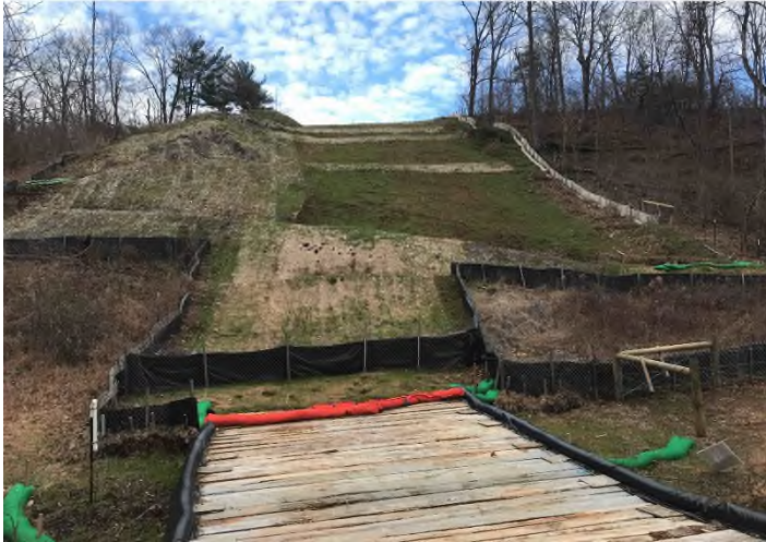
Figure 3: Stream S-GH9 – Controls in place and functioning properly. Area stabilized with erosion matting. No evidence of sediment discharge off ROW.
