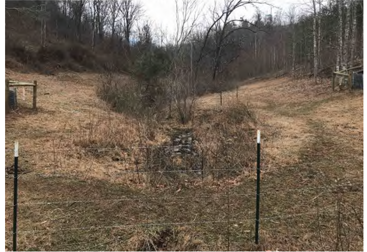
Figure 4: Stream S-GH9 – Controls in place and functioning properly. Area stabilized with erosion matting. No evidence of sediment discharge off ROW.
