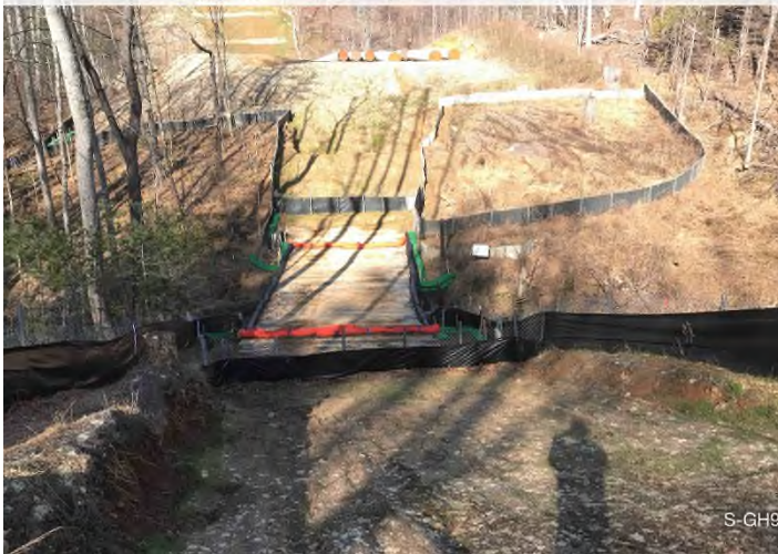
Figure 3: Stream S-GH9 – Controls in place and functioning properly. Area stabilized with erosion matting. No evidence of sediment discharge off ROW.
