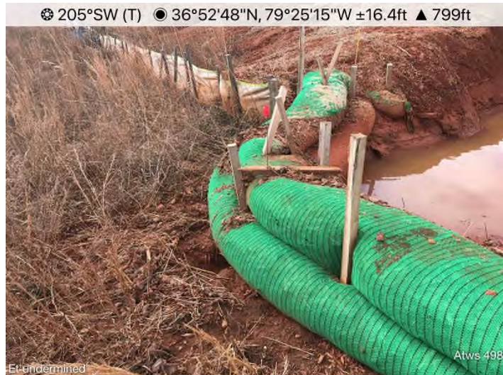
Figure 3: ATWS 498 – End treatment CFS undermined. Maintenance needed.
