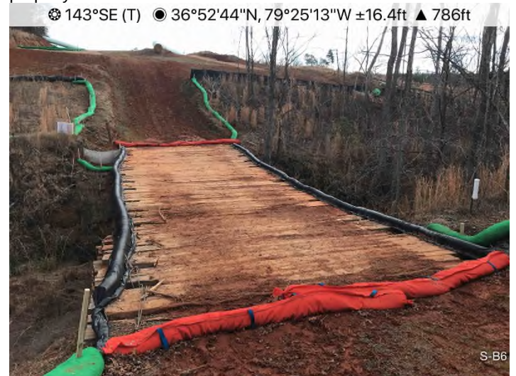
Figure 4: Stream S-B6 – Controls in place and functioning properly.
