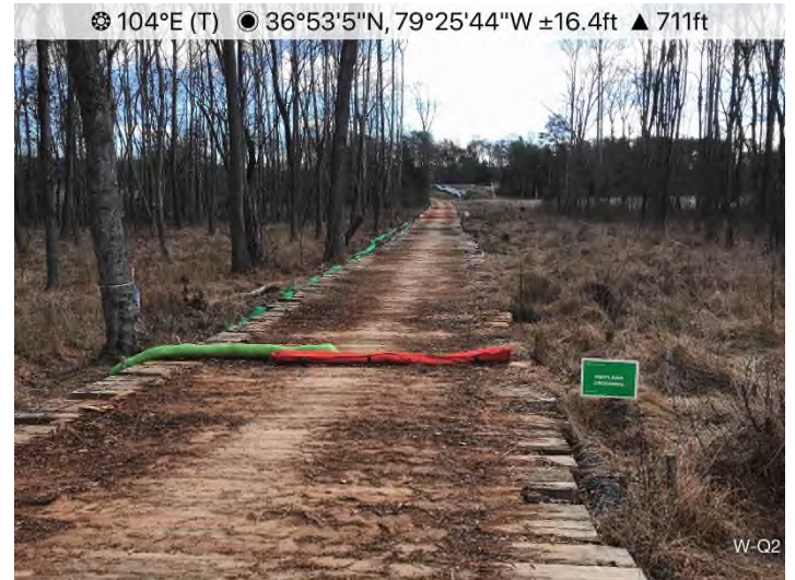
Figure 4: Stream S-B6 – Controls in place and functioning properly.
