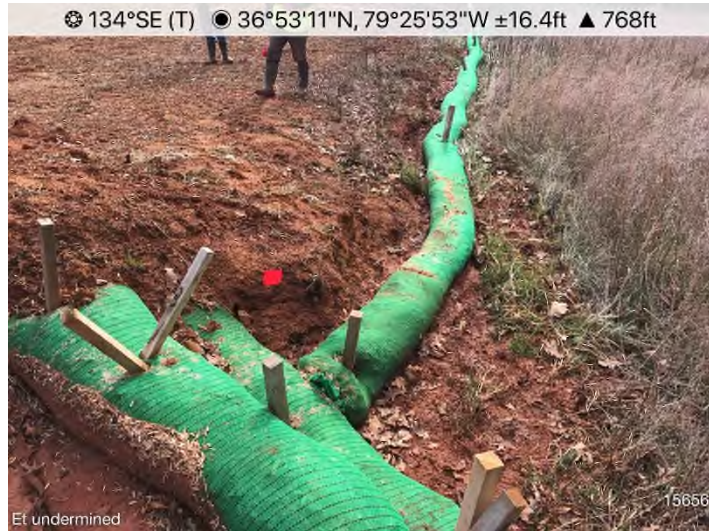
Figure 3: ATWS 498 – End treatment CFS undermined. Maintenance needed.
