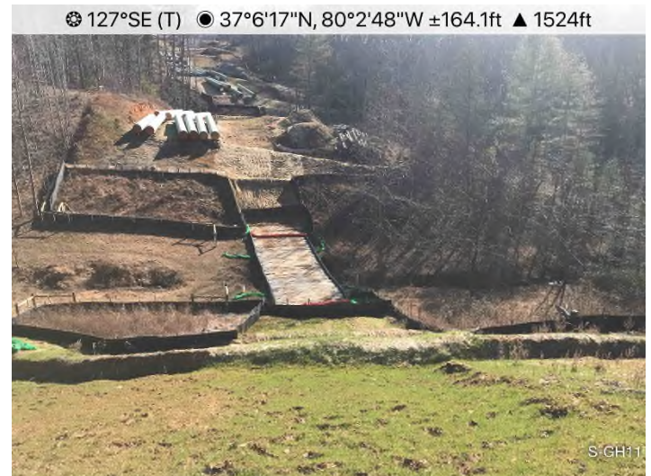
Figure 4: STA 13333+00 – Controls in place and functioning properly above Stream S-GH11.
