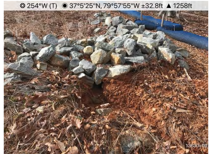
Figure 4: STA 13629+45 – Permanent end-treatment level spreader undermined. Repair needed.
