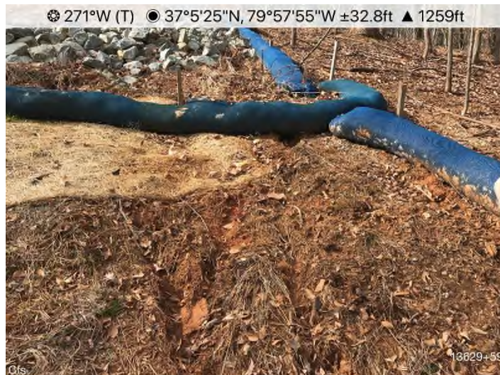
Figure 3: STA 13629+50 – CFS undermined. Maintenance needed.
