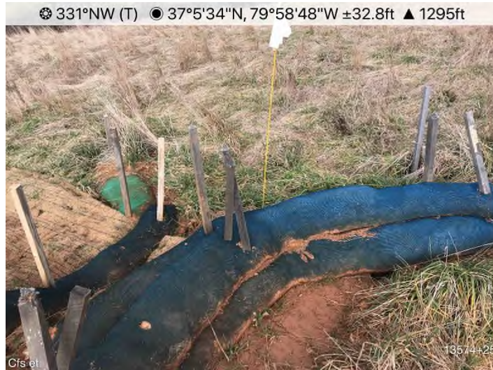
Figure 3: STA 13629+50 – CFS undermined. Maintenance needed.
