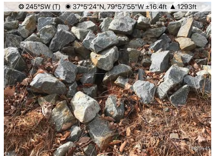
Figure 4: STA 13629+45 – Permanent end-treatment level spreader undermined. Repair needed.
