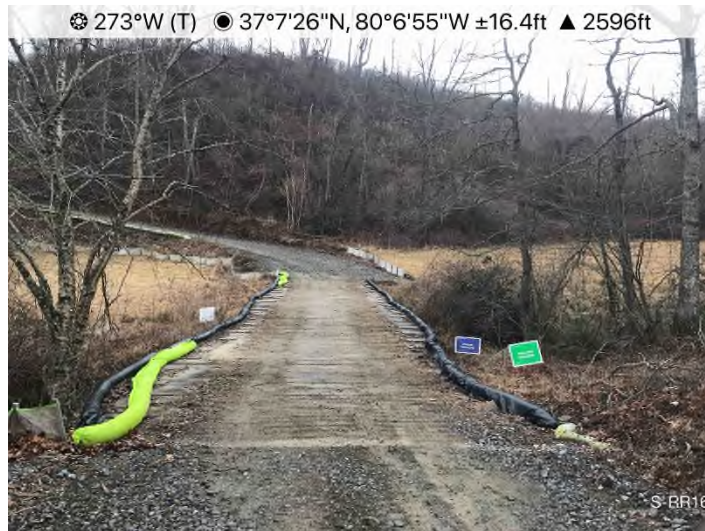
Figure 3: Stream S-NN16 – Controls in place and functioning properly around the Roanoke River.
