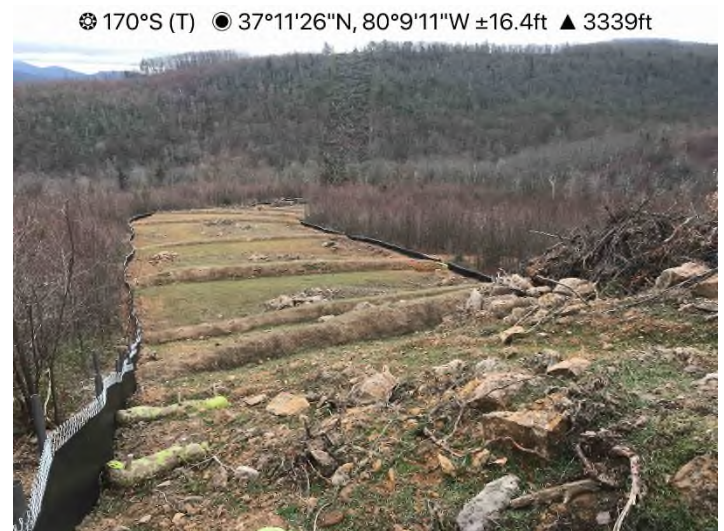
Figure 4: ATWS 727 – Controls in place and functioning properly. Area stabilized with vegetation.
