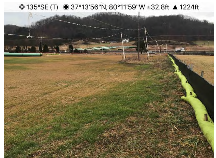
Figure 4: ATWS 727 – Controls in place and functioning properly. Area stabilized with vegetation.
