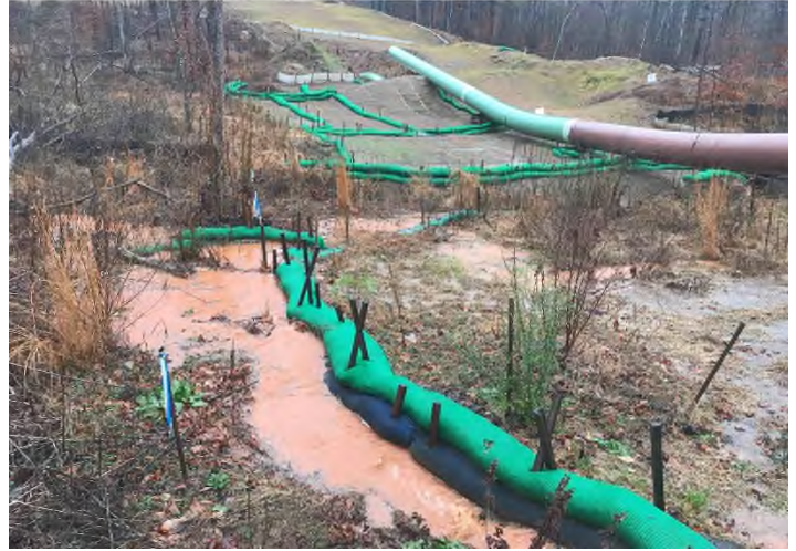
Figure 4: STA 14233+50 – Maggodee Creek crossing looking W. Controls in place and functioning properly.
