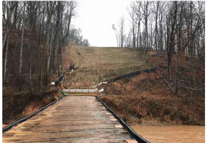
Figure 4: STA 14233+50 – Maggodee Creek crossing looking W. Controls in place and functioning properly.
