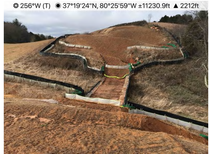
Figure 16: STA 11480+00 – No offsite sediment discharge evident above karst “sinkhole” feature.
