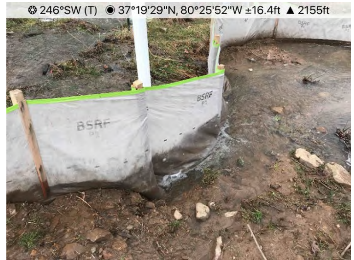
Figure 8: STA 11489+80 – Perimeter P1 undermined due to onsite run-on from stream S-PP2.
