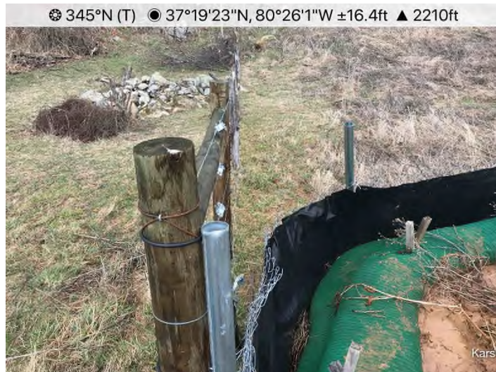
Figure 15: STA 11480+50 – Controls in place and functioning properly above “sinkhole”. No offsite sediment discharge evident.
