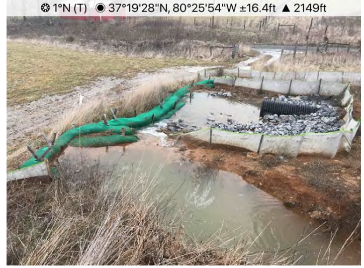
Figure 12: STA 11488+50 – Waterbar end-treatment overwhelmed. Discharge entering CWD. STA 11489+00 CWD end-treatment undermined.
