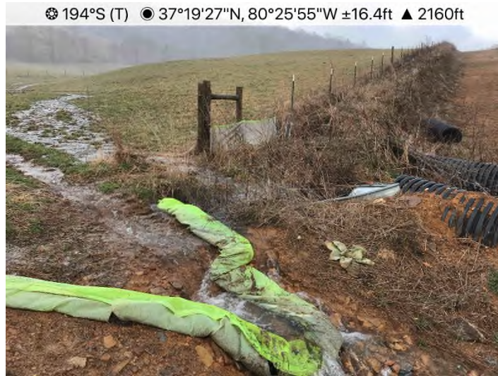
Figure 11: STA 11488+50 – Offsite storm water run-on flowing down waterbar.
