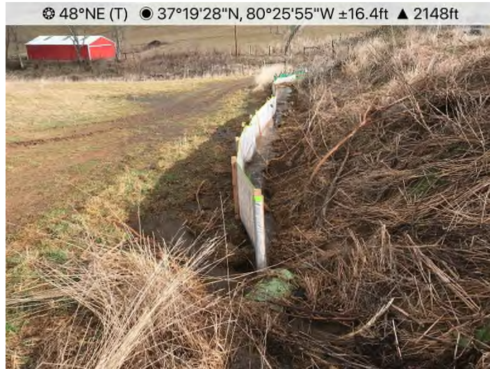
Figure 15: STA 11480+50 – Controls in place and functioning properly above “sinkhole”. No offsite sediment discharge evident.
