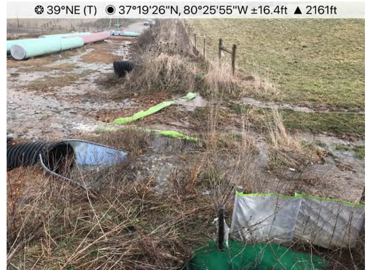
Figure 12: STA 11488+50 – Waterbar end-treatment overwhelmed. Discharge entering CWD. STA 11489+00 CWD end-treatment undermined.
