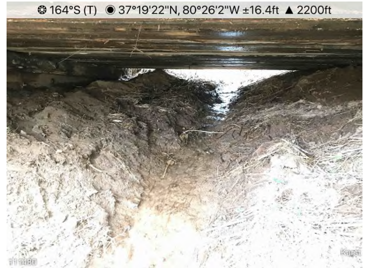
Figure 18: STA 11480+00 – Stabilize denuded drainage channel under bridge crossing.
