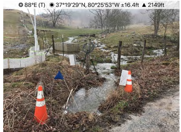
Figure 8: STA 11489+80 – Perimeter P1 undermined due to onsite run-on from stream S-PP2.
