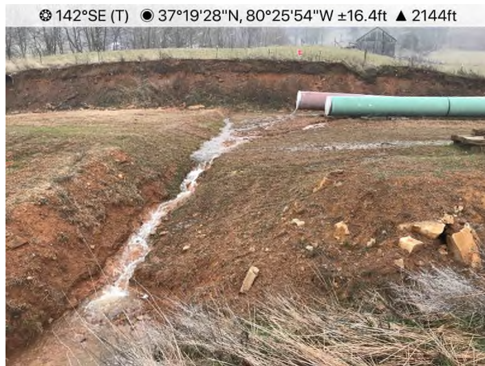
Figure 11: STA 11488+50 – Offsite storm water run-on flowing down waterbar.
