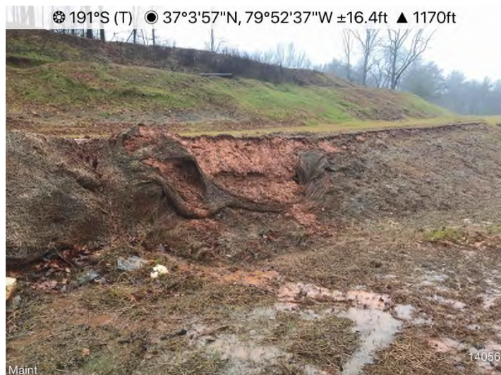
Figure 3: STA 14056+00 – Erosion matting repair needed.
