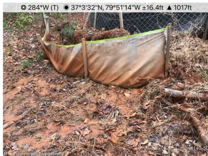
Figure 8: STA 14142+30 – CFS undermined. Maintenance needed.
