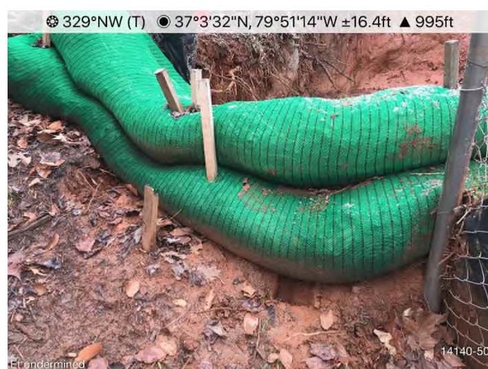
Figure 4: STA 14140+50 – End Treatment undermined. Maintenance needed.
