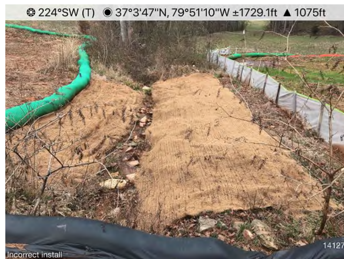
Figure 4: STA 14140+50 – End Treatment undermined. Maintenance needed.
