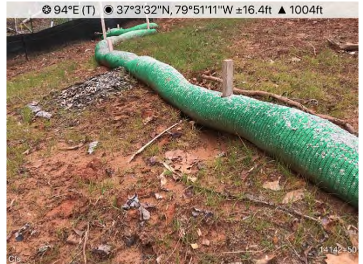
Figure 12: STA 14144+50 – Sediment off ROW. Retrieve and stabilize sediment.
