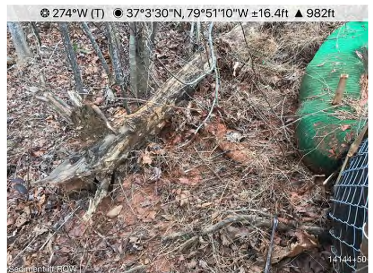
Figure 12: STA 14144+50 – Sediment off ROW. Retrieve and stabilize sediment.
