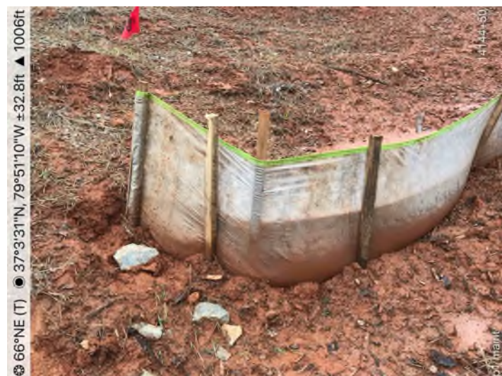
Figure 15: STA 14150+00 – End Treatment undermined. Maintenance needed.
