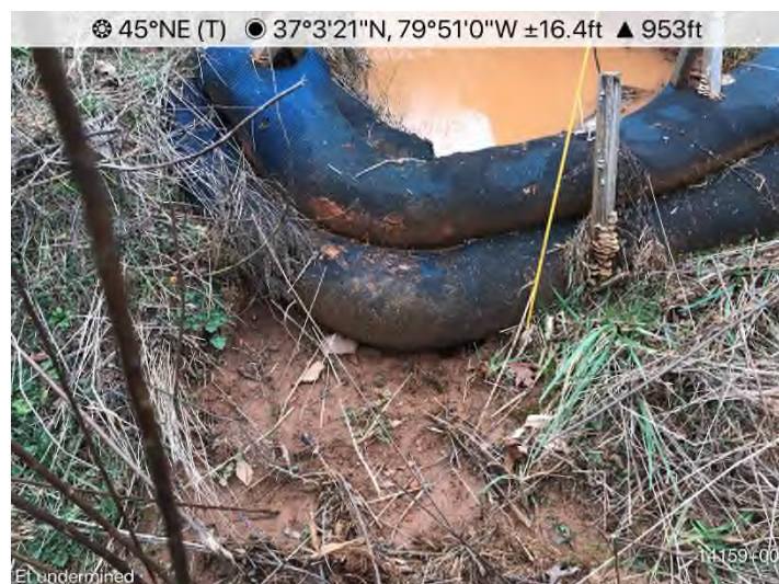
Figure 15: STA 14150+00 – End Treatment undermined. Maintenance needed.
