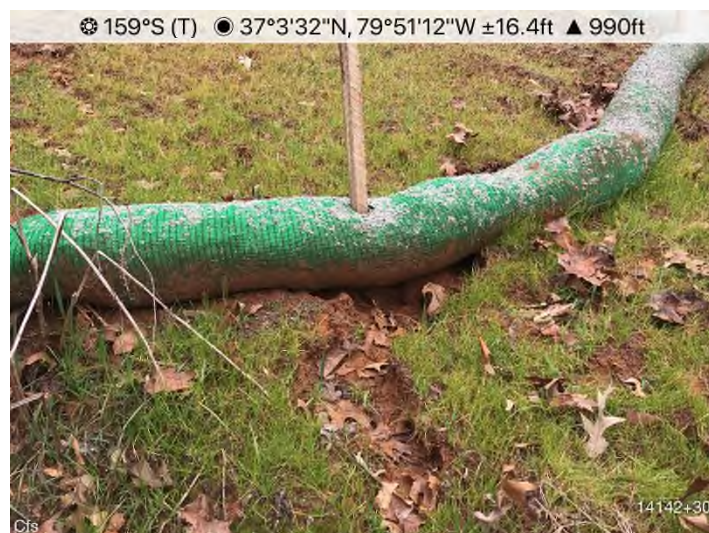
Figure 8: STA 14142+30 – CFS undermined. Maintenance needed.
