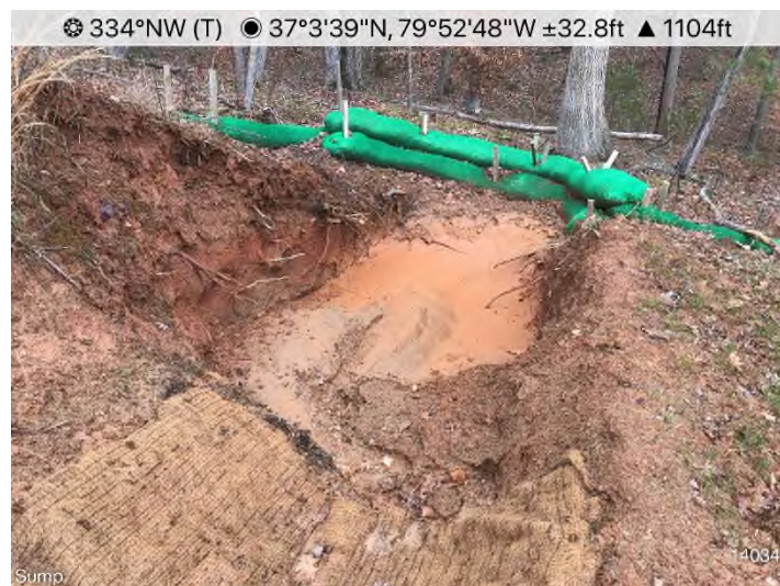
Figure 3: STA 14140+00 – CFS maintenance needed.
