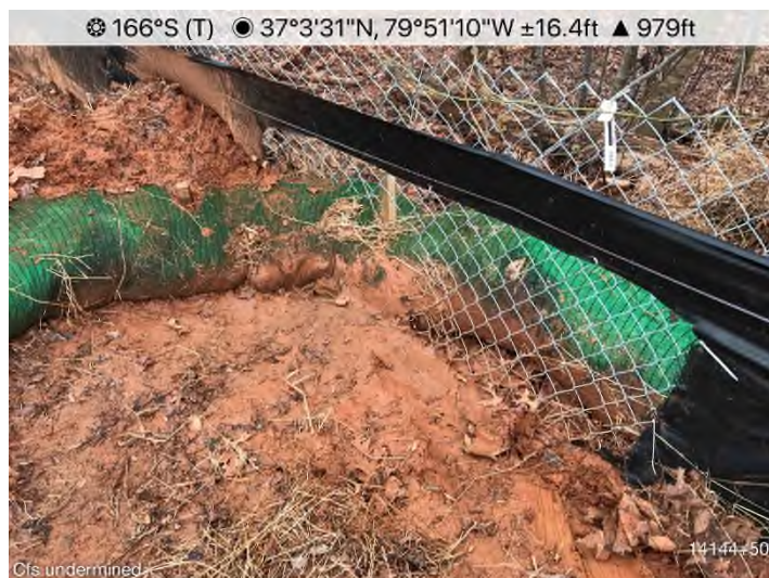
Figure 11: STA 14144+50 – CFS undermined. Maintenance needed.
