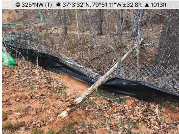
Figure 11: STA 14144+50 – CFS undermined. Maintenance needed.
