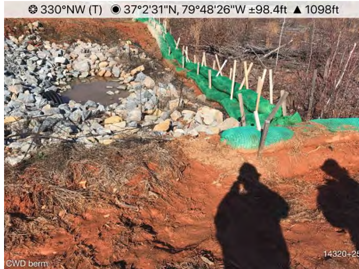
Figure 3: STA 14320+25 – Plunge pool diversion berm repair needed.
