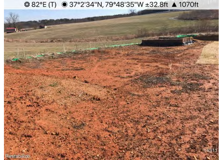
Figure 4: STA 14320+25 – Re-stabilization needed.
