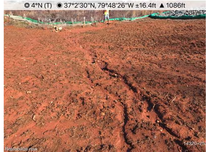
Figure 4: STA 14320+25 – Re-stabilization needed.
