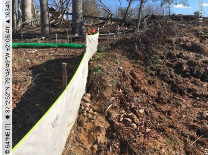
Figure 3: STA 14320+25 – Plunge pool diversion berm repair needed.
