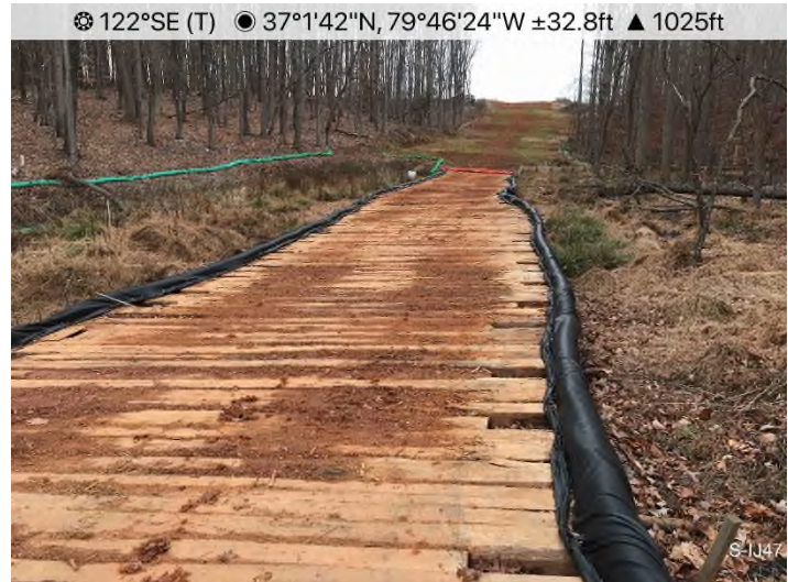
Fig. 4: STA 14480+50 – Controls in place and functioning properly around Stream S-G22.
