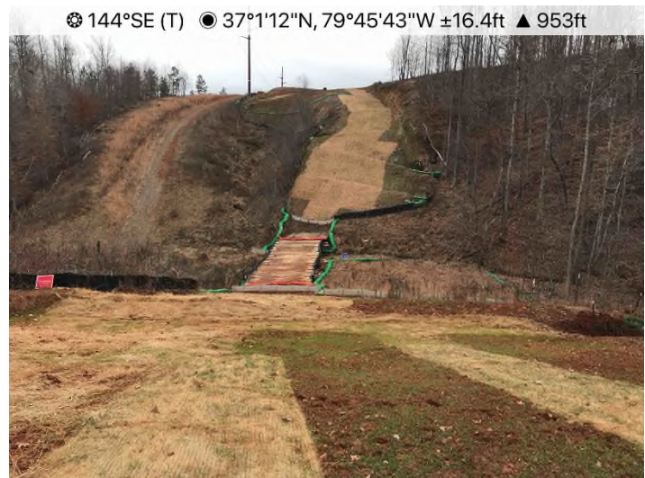
Fig. 4: STA 14480+50 – Controls in place and functioning properly around Stream S-G22.
