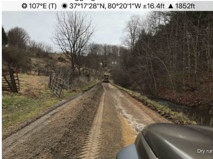
Fig. 11: Dry Run Road – VDOT repairing Dry Run Road from Catawba Rd. to Mt. Tabor Rd. Rain event caused significant erosion to road along Dry Run depositing sediment and road aggregate into stream.
