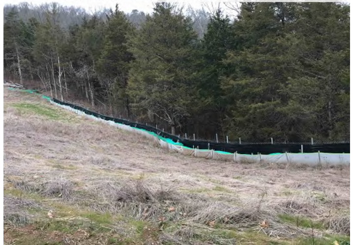
Fig. 4: STA 11978+00 – Controls in place above karst feature on the east of ROW. Area stabilized with vegetative cover. No erosion evident.
