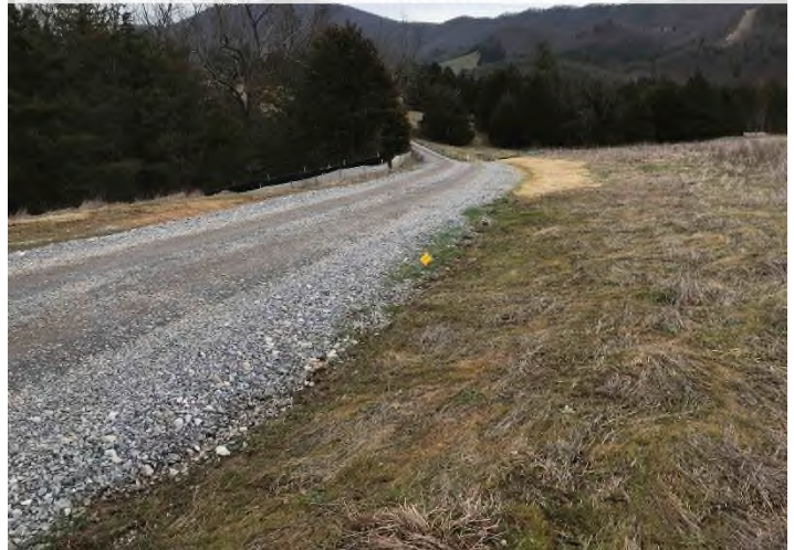
Fig. 4: STA 11978+00 – Controls in place above karst feature on the east of ROW. Area stabilized with vegetative cover. No erosion evident.
