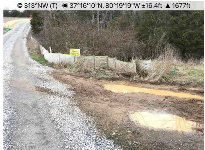
Fig. 12: Catawba Road Crossing – Controls in place and functioning at Catawba Road.
