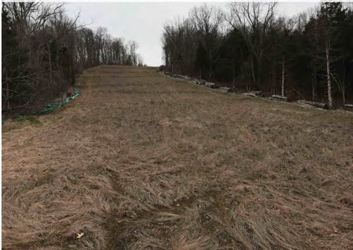
Fig. 3: STA 11977+00 – Looking north towards underground gravel filter bed. Controls in place. Area stabilized with vegetative cover. No erosion evident.
