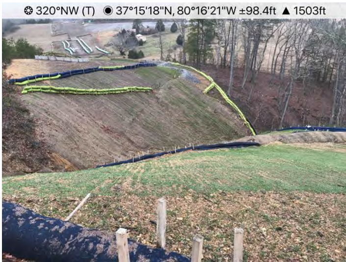
Fig. 3: STA 12147+00 – Controls in place and functioning properly. Area stabilized.
