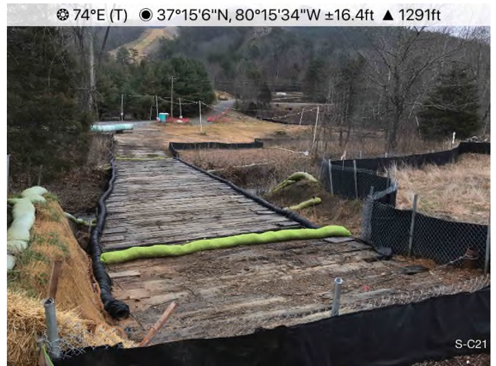
Fig. 4: STA 12192+00 – Controls in place above Stream S-C21 Bradshaw Creek.
