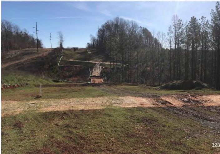
Fig. 3: STA 14802+00 – Controls in place and functioning properly. Area stabilized with vegetation and Earth Guard.
