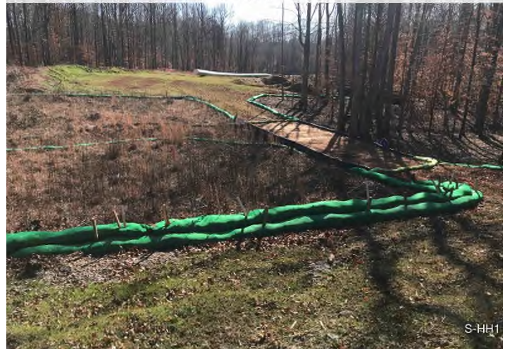
Fig. 4: Stream S-HH1 – Controls in place and functioning properly. Area stabilized with vegetation.
