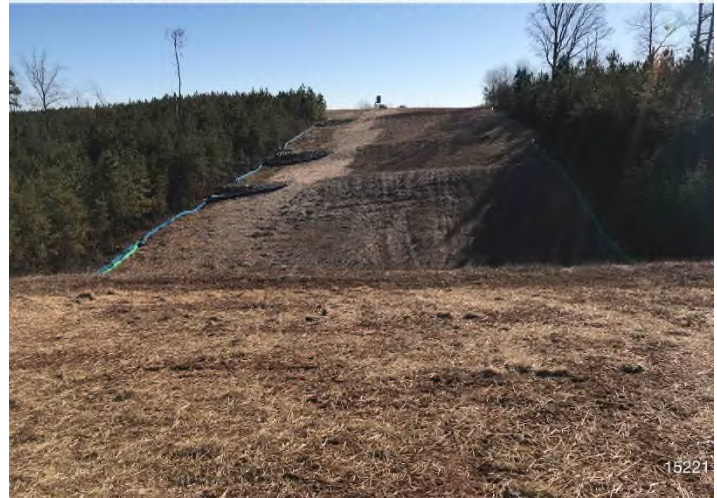
Fig. 4: Stream S-HH1 – Controls in place and functioning properly. Area stabilized with vegetation.
