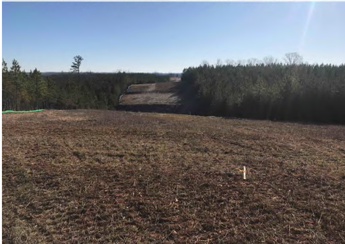
Fig. 3: STA 14802+00 – Controls in place and functioning properly. Area stabilized with vegetation and Earth Guard.
