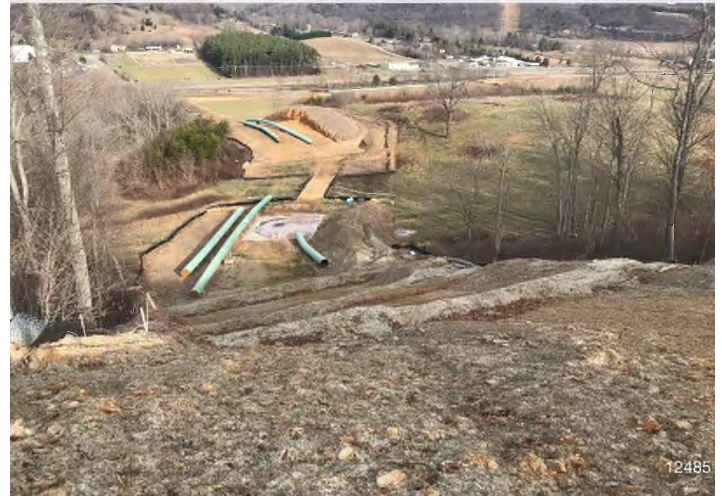
Figure 4: STA 12485+00 – Controls in place and functioning properly. Area stabilized with straw, hydro-mulch and erosion matting.
