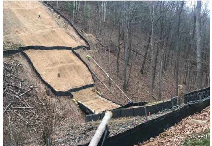
Figure 4: STA 12485+00 – Controls in place and functioning properly. Area stabilized with straw, hydro-mulch and erosion matting.
