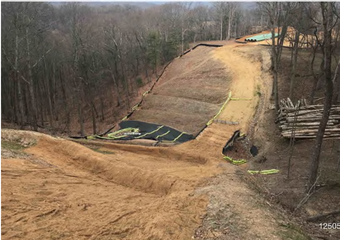
Figure 3: STA 12505+00 – Controls in place and functioning properly. Area stabilized with straw, hydro-mulch and erosion matting.
