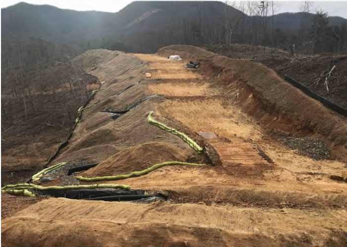
Figure 3: STA 12505+00 – Controls in place and functioning properly. Area stabilized with straw, hydro-mulch and erosion matting.
