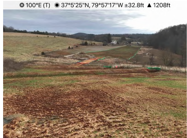
Fig. 4: STA 13738+00 – Controls in place and functioning properly. Area stabilized with Flexterra.
