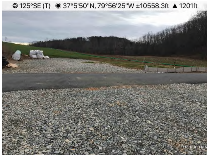
Fig. 3: STA 13727+50 – Controls in place around Stream S-EF4 crossing. Area stabilized.
