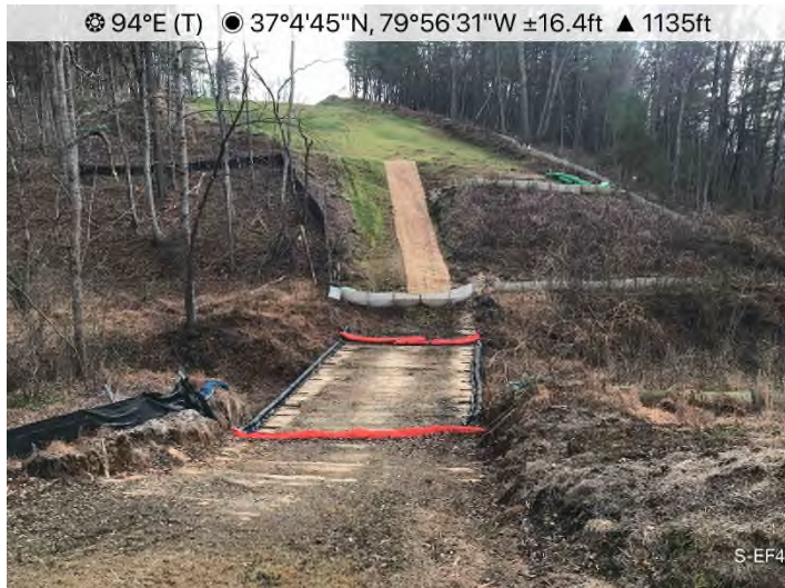
Fig. 3: STA 13727+50 – Controls in place around Stream S-EF4 crossing. Area stabilized.
