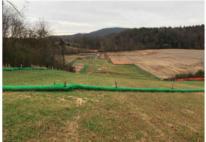
Fig. 4: STA 13906+50 – Controls in place and functioning properly. Area stabilized.
