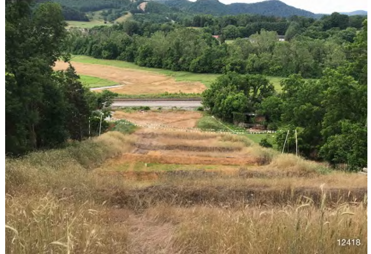
Figure 4: STA 12385+00 – Controls in place and functioning properly. Area stabilized.
