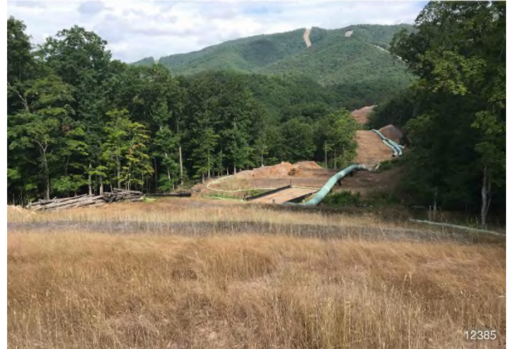
Figure 4: STA 12385+00 – Controls in place and functioning properly. Area stabilized.
