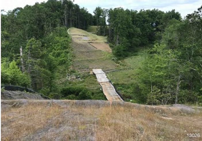
Figure 3: STA 13026+00 – Controls in place and functioning properly. Area stabilized with vegetation and erosion control fabric.
