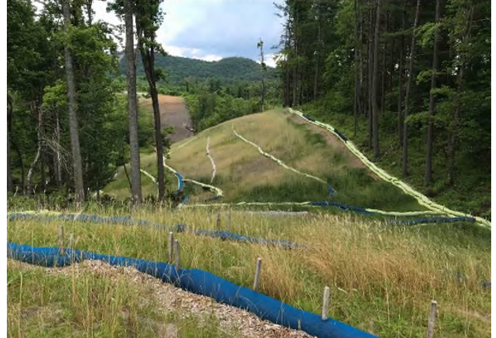
Figure 4: STA 13020+00 – Controls in place and functioning properly. Area stabilized.
