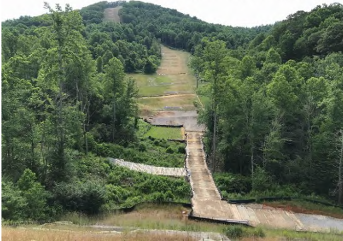
Figure 3: STA 13026+00 – Controls in place and functioning properly. Area stabilized with vegetation and erosion control fabric.
