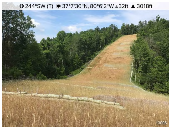
Figure 3: STA 13098+00 – Controls in place and functioning properly. Area stabilized.
