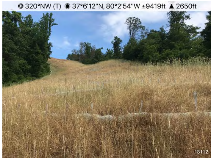
Figure 3: STA 13098+00 – Controls in place and functioning properly. Area stabilized.
