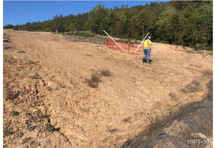
Figure 4: STA 12171+00 – Controls in place and functioning properly. Area stabilized with erosion matting and straw.
