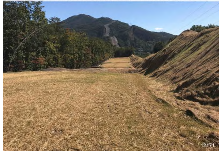
Figure 4: STA 12171+00 – Controls in place and functioning properly. Area stabilized with erosion matting and straw.
