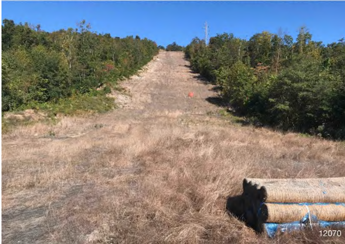
Figure 3: STA 12153+00 to 12154+00 – Re-stabilization needed.
