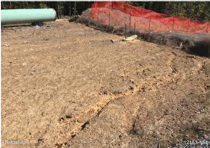
Figure 3: STA 12153+00 to 12154+00 – Re-stabilization needed.
