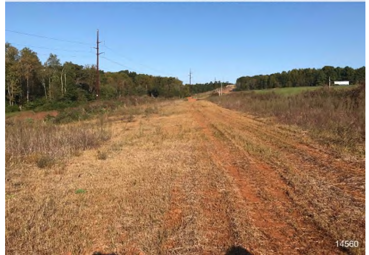
Figure 4: STA 14572+00 – Controls in place and functioning properly. Area stabilized with straw.
