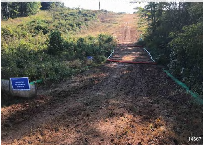
Figure 3: STA 14567+00 – Controls in place and functioning properly. Area stabilized with straw.
