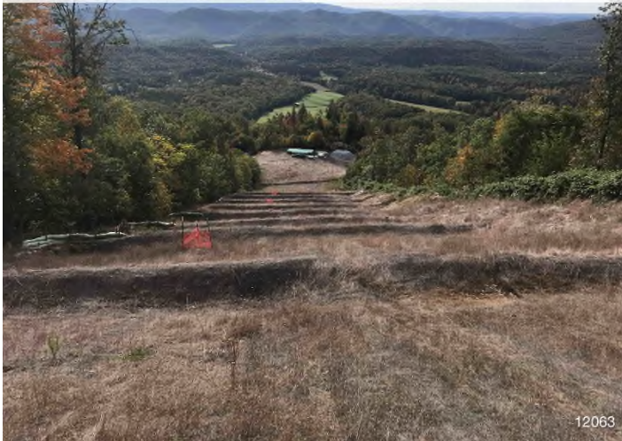
Figure 3: MVP-MN-268.01 – PPL crews installing erosion control matting and applying temporary seed along MN-268.01.
