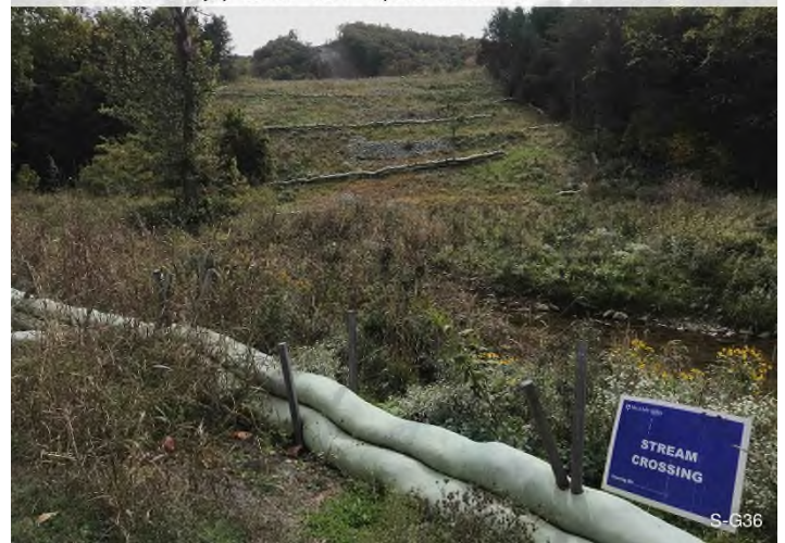
Figure 4: Stream S-G36 – Controls in place and functioning properly around N. Fork Roanoke River crossing.
