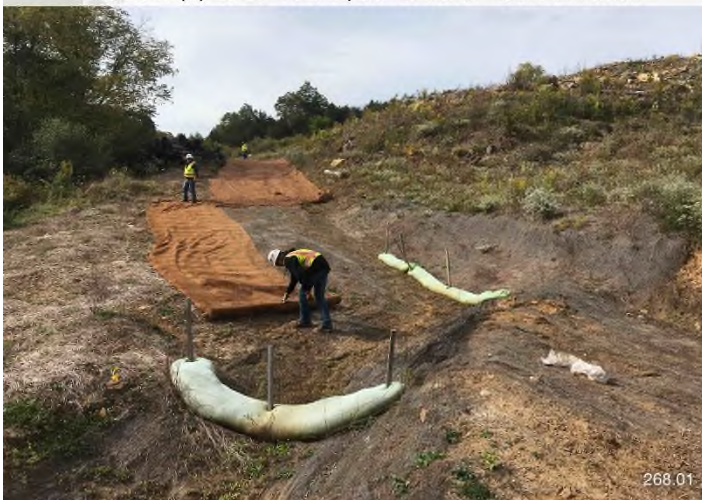
Figure 3: MVP-MN-268.01 – PPL crews installing erosion control matting and applying temporary seed along MN-268.01.
