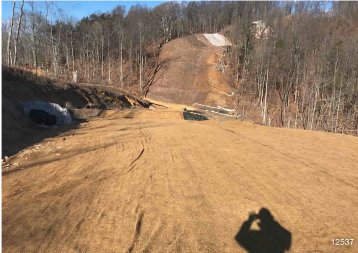
Figure 1: STA 12537+00 – Controls in place and functioning properly. Area Stabilized with straw and erosion control fabric. BRG: 312°NW (T) LAT: 37.211547 LON: -80.195502 ±98ft ALT: 1681ft
