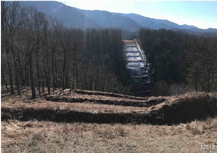
Figure 3: STA 12513+00 – Controls in place and functioning properly. Area Stabilized with straw and erosion control fabric. BRG: 178°S (T) LAT: 37.217770 LON: -80.197356 ±32ft ALT: 1934ft
