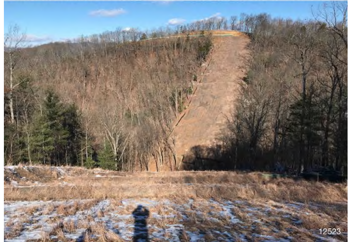
Figure 2: STA 12523+00 – Controls in place and functioning properly. Area Stabilized with straw and erosion control fabric. BRG: 355°N (T) LAT: 37.197756 LON: -80.233750 ±9843ft ALT: 1787ft
