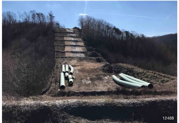
Figure 4: STA 12488+00 – Controls in place and functioning properly. Area Stabilized with straw and erosion control fabric. BRG: 156°SE (T) LAT: 37.226162 LON: -80.203033 ±8067ft ALT: 1537ft
