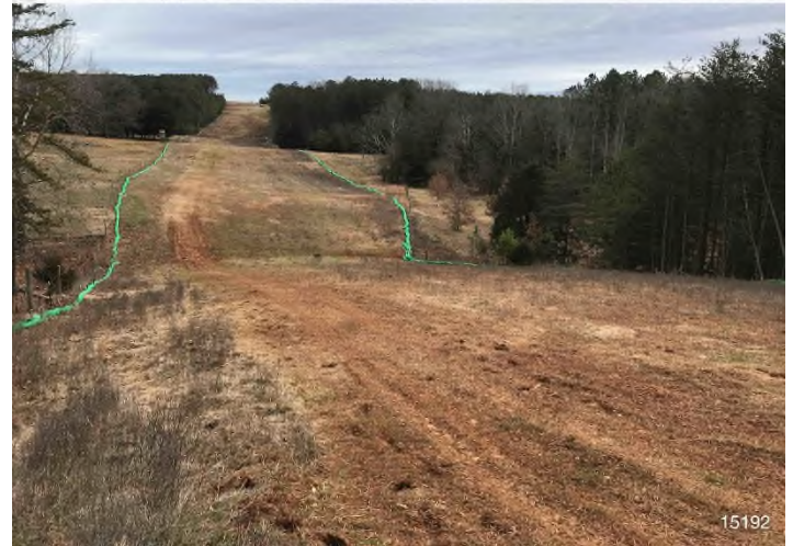
Figure 4: STA 15192+00 – Controls in place and functioning properly. Area stabilized with straw.
