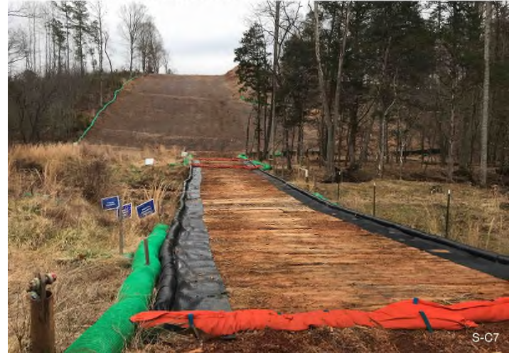
Figure 4: STA 15192+00 – Controls in place and functioning properly. Area stabilized with straw.
